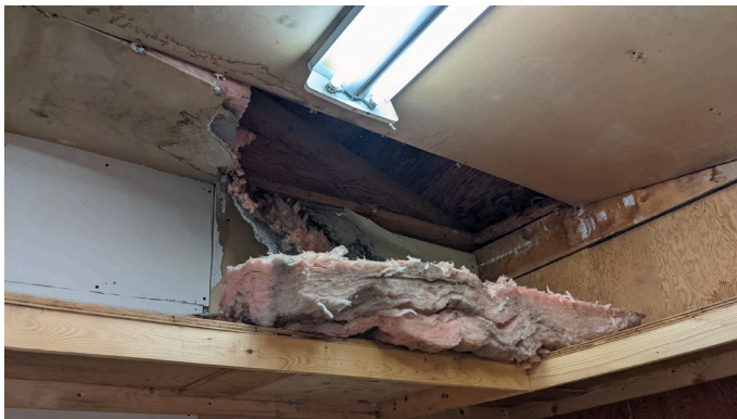
Photo 12: Water Damage & Insulation
