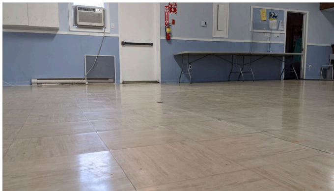
Photo 8: Uneven Floor Indicating Floor Joist Damage
