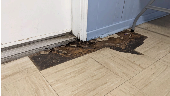
Photo 7: Courtyard Door Water Infiltration
