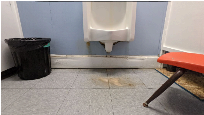
Photo 9: Male Washroom Floor Damage
