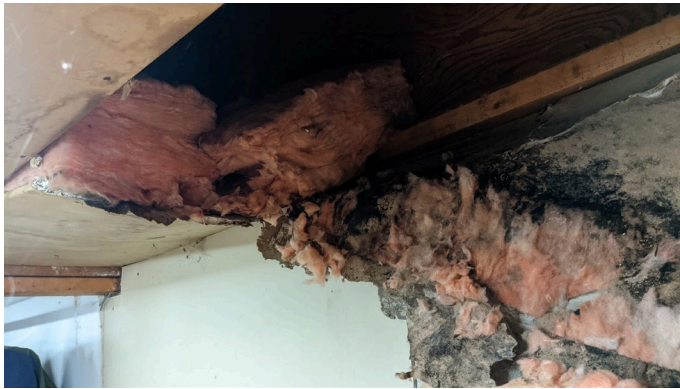
Photo 14: Water & Ceiling Damage
