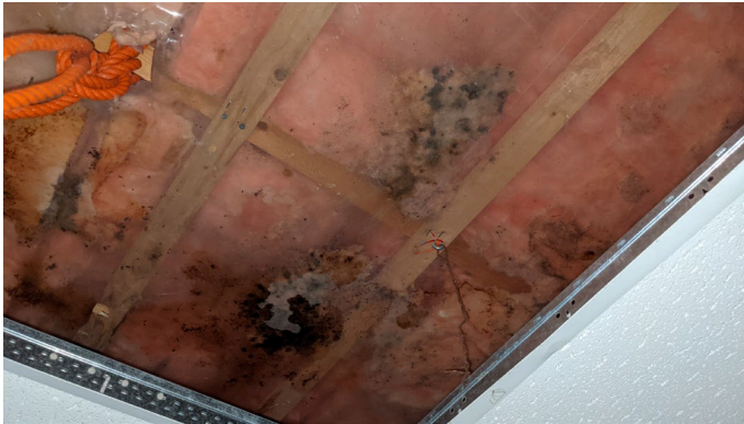
Photo 12: Water Damage & Insulation
