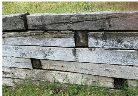
Treated wood retaining wall
