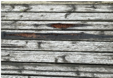
Treated wood walkway
