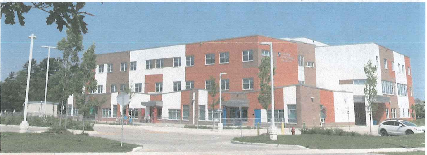
Figure 14 - Hyde Park School, Barrie by S+A - awarded the most energy efficient school in North America
